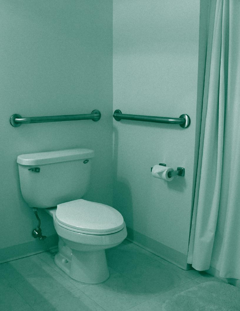
**If you hit a stud (indicated by wood shaving after penetrating the dry wall material):** Stop drilling. Change to a 1/8" drill bit and finish drilling a pilot hole into the stud. The hole should now be ready for use with a long wood screw. The best choice is a stainless steel wood screw that is as long as possible (up to 4 inches) with a pan head.
